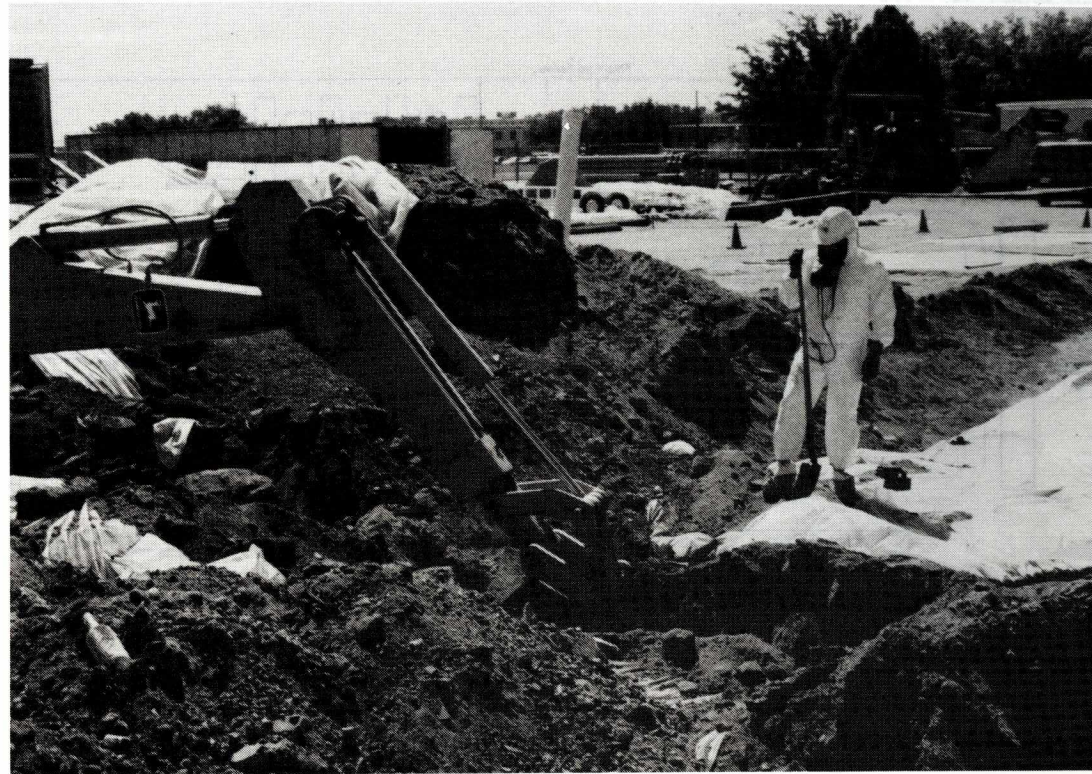
Figure 6. Heavy equipment was used to open one of the sample trenches archaeologists used to study the deposits in the first Proving Ground Dump.
