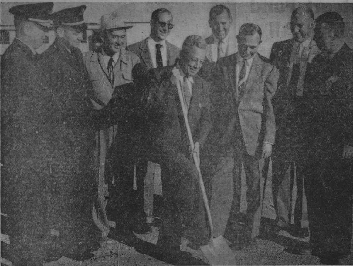
DIGGING FOR A DREAM — In ground-breaking ceremonies, Flight Simulation Laboratory Chief Guenther Hintze turns over the first spadeful of dirt for his new laboratory building. Watching the operation, from left, are Lt. Col. John G. Redmon and Capt. C. W. Kingsbury of Ordnance Mission; J. S. Wilborn, resident engineer; R. W. Hutchinson, personnel officer; Construction Supt. J. W. Cadwell; V. M. Capos, construction engineer; A. O. Crobaugh, chief of Electro-Mechanical Laboratories, and Warren J. Brown, physicist. Cadwell and Cobbs are in charge of the project for the Robert E. McKee Co. of El Paso, which won the contract with a bid of $610,440.
